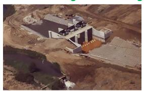
In 1982, the then-Southern Water Authority finished constructing the Leigh Flood Storage Area (FSA) to reduce the risk of flooding to approximately 1,200 homes and businesses in Tonbridge and Hildenborough. The FSA works to store the peak of a flood upstream and release it in a controlled manner once the peak has passed.
